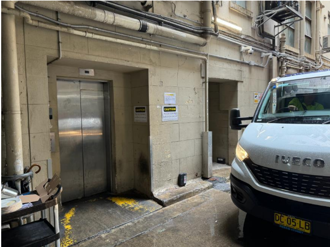
Figure 15: Lift with access to lower levels adjoining Parlour Lane
