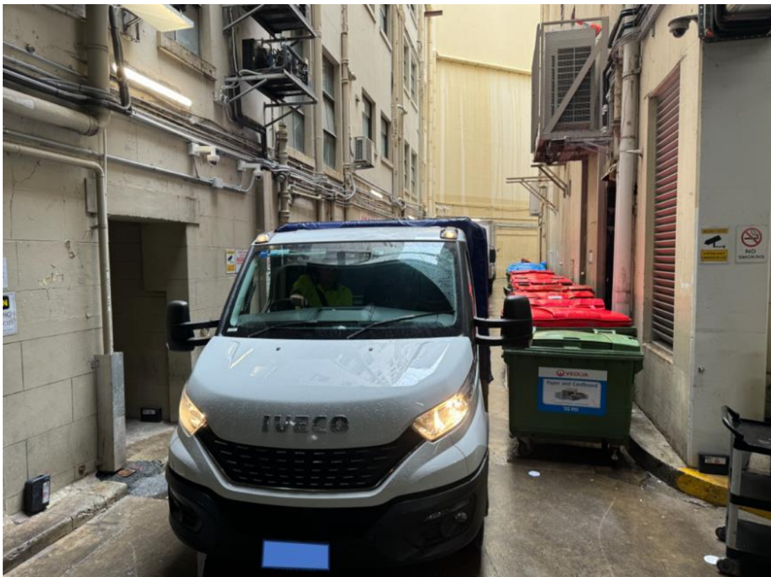
Figure 16: Parlour Lane along the western side of the State Theatre, including waste storage
